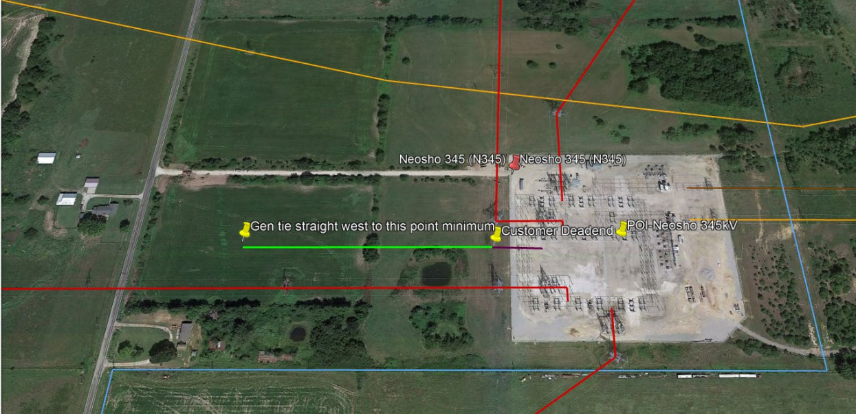
Figure 1 –Neosho 345kV Substation
